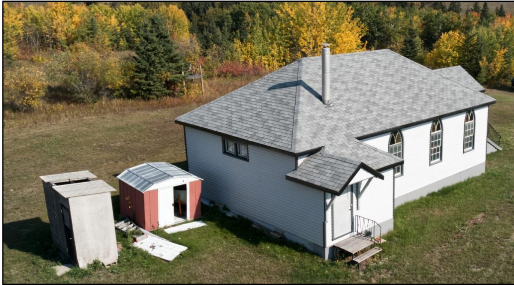
Asking for trouble: ladders, unlocked shed with lawnmower and gasoline.
